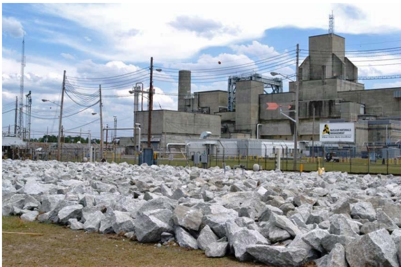
Figure 4. Rip Rap Outside the Perimeter Intrusion Detection and Assessment System to Impair Adversary Movement
