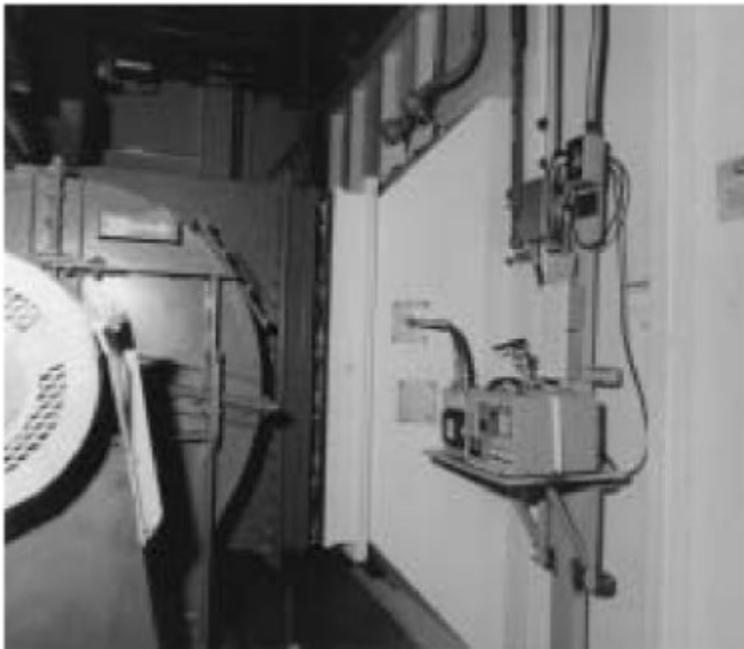
**Figure 4.69: Air Monitor in Exhaust Duct from Plenum**
