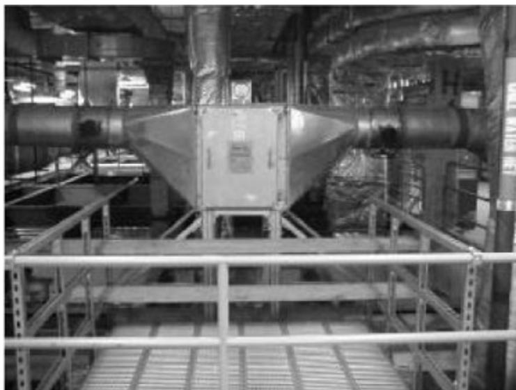
**Figure 4.24: Correct Mounting of In-Duct-HEPA Filter Housing**
