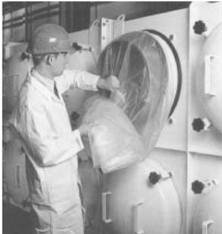
**Figure 4.74: Radial Flow Filter Bag-Out**
