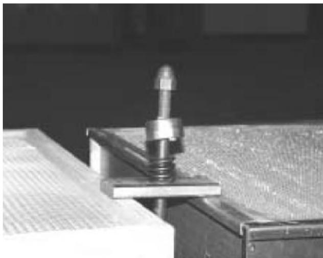
**Figure 4.55: Filter Hold-Down (Spring Design)**
