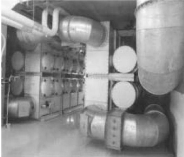
**Figure 4.73: Side Access Housing**
