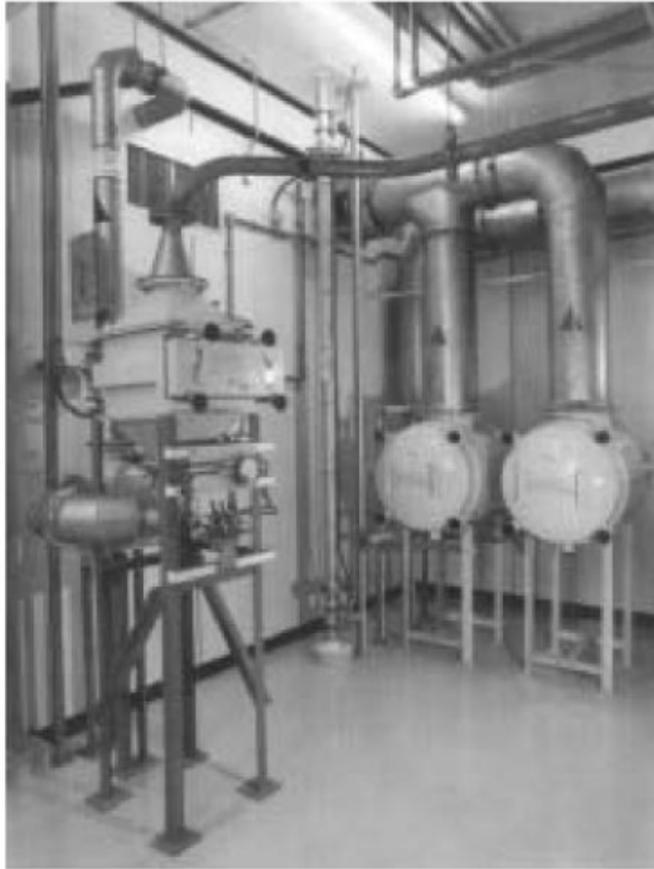
**Figure 4.71: Side-Access Housing**
