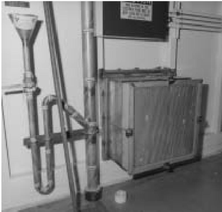
Figure 4.63: Filter Plenum Drain P-Trap Fill Tube
