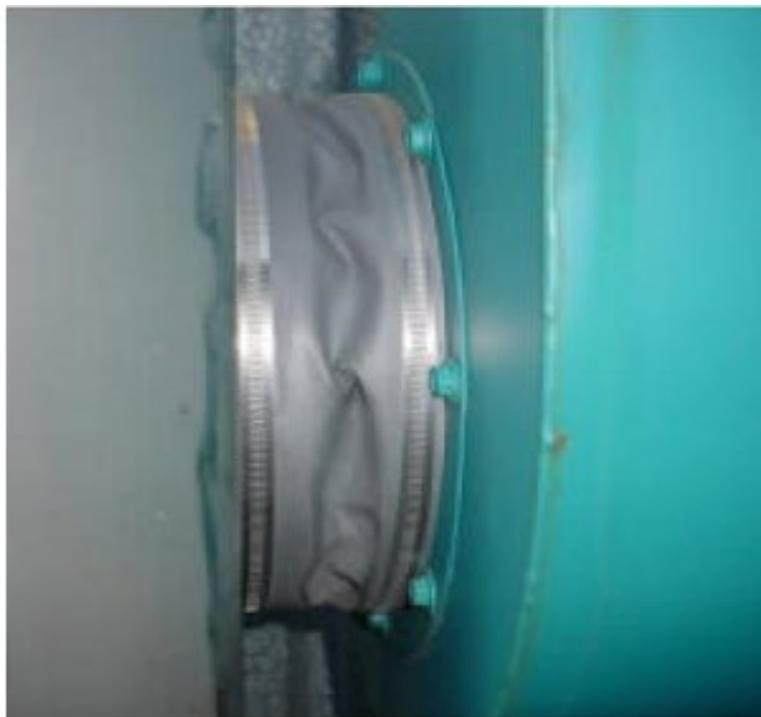
**Figure 4.34: Flexible Connection**
