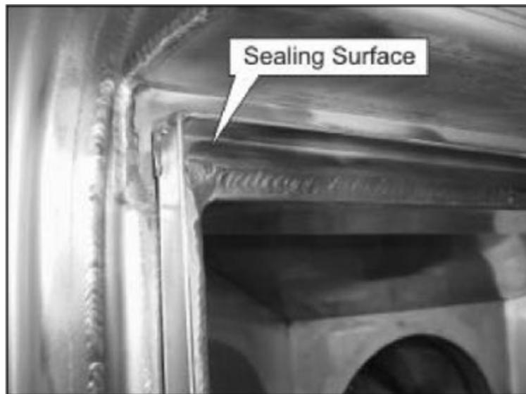
**Figure 4.28: Gel Seal Commercial Housing Filter Sealing Surface**
