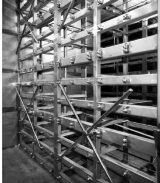
Figure 8.16 – Adsorber Tray Mounting Frame. “X” Cross Units Are for Test Gas Injection
