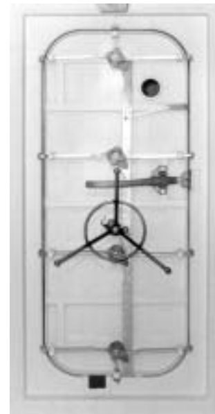
Figure 4.52 – Plenum Door (Wheel-Type Inside Plenum Access)
