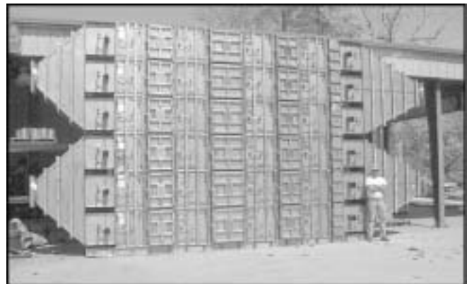
Figure 4.55 – Side Access Housing with Combination of Filter and Adsorber Sections
