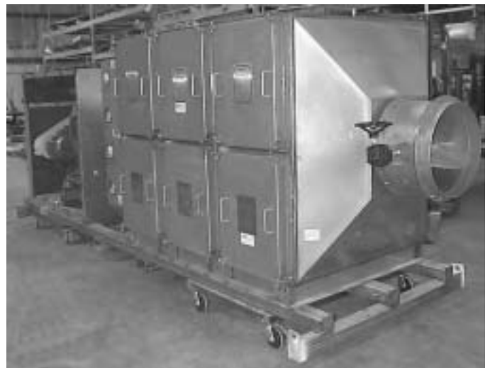
Figure 4.59 – Side-Access Housing with Single Air Entry
