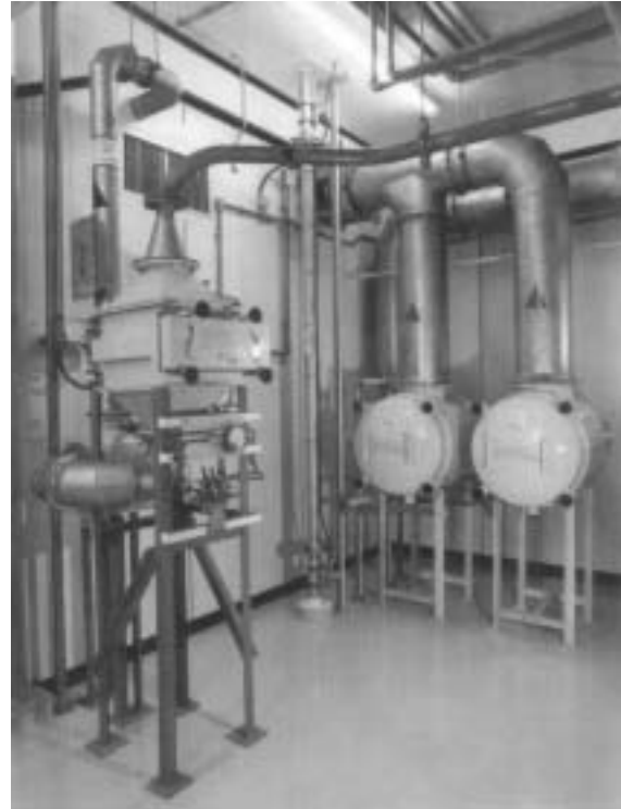
Figure 4.68 – Side-Access Housing (Cylindrical Radial Flow HEPA Design)
