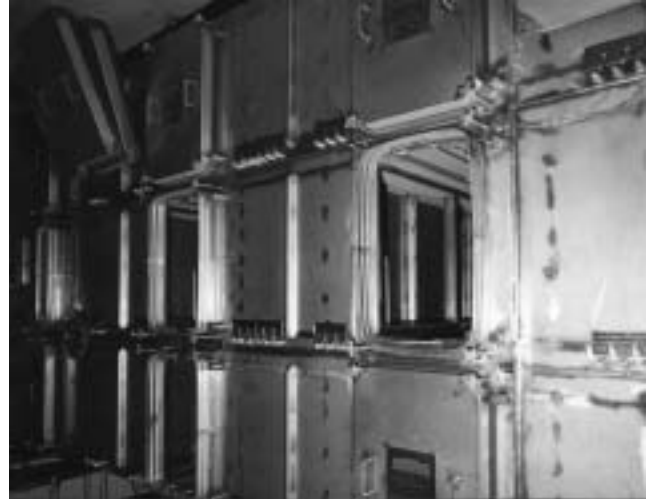
Figure 4.53 – Bag-In/Bag-Out Filter Housing
