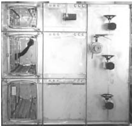
Figure 4.64 – Side-Access Housing
