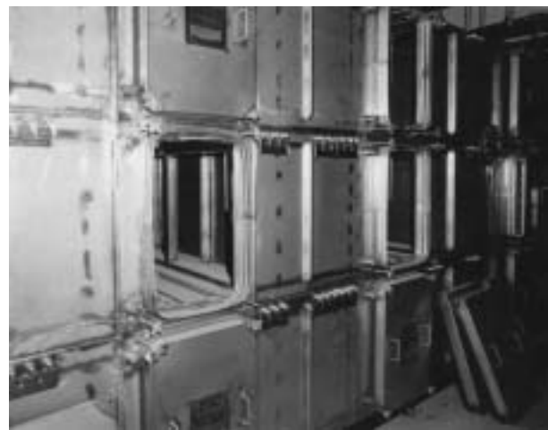
Figure 4.65 – Side Access-Housing with Bag-In/Bag-Out Covers
