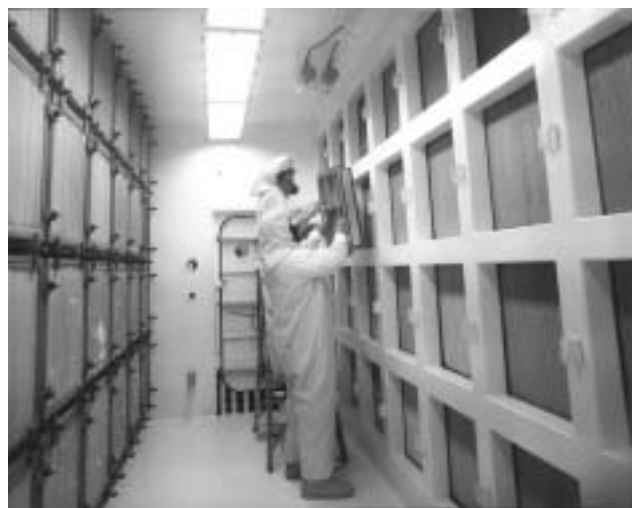
Figure 4.30 – Blanking Plate Being Installed On Downstream Side of Mounting Frame
