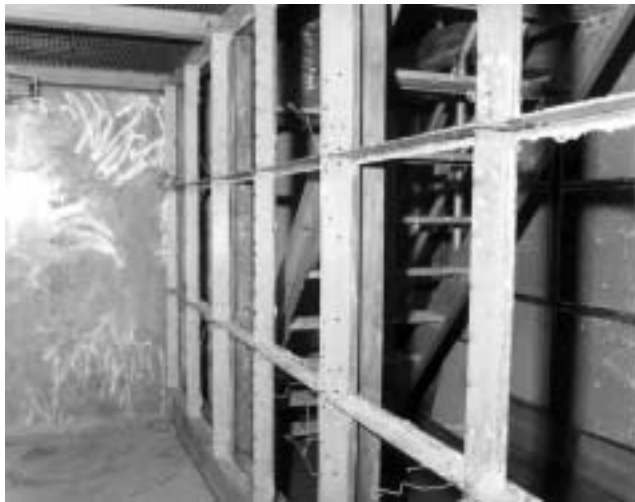
Figure 4.42 – Moisture Separator Mounting Frame
