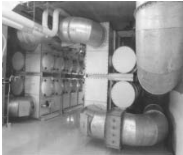
Figure 4.70 – Side-Access Housing (Cylindrical Radial Flow HEPA Design)
