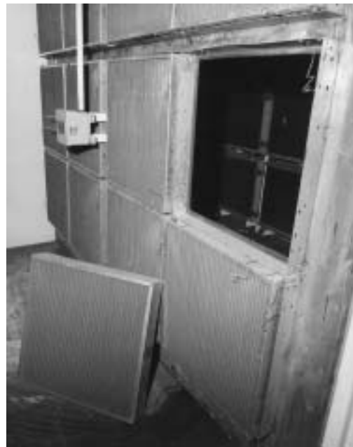
Figure 4.43 – Moisture Separator and Mounting Frame
