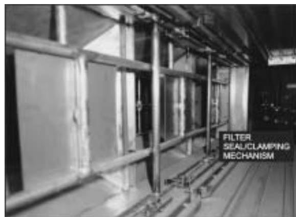
Figure 4.67 – Side-Access Housing with Test Manifold
