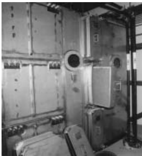
Figure 4.66 – Side-Access Housing with Moisture Separator
