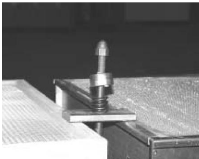
Figure 4.55: Filter Hold-Down (Spring Design)
