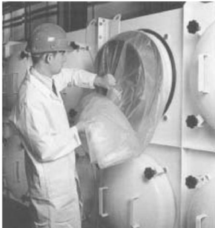
Figure 4.74: Radial Flow Filter Bag-Out
