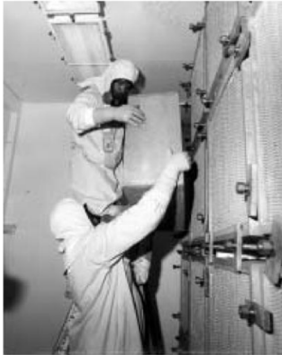
Figure 4.58: HEPA Filter Mounted on Upstream Side of Mounting Frame Filter Replacement
