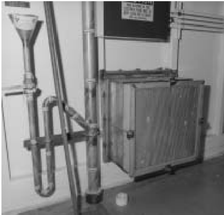
Figure 4.63: Filter Plenum Drain P-Trap Fill Tube
