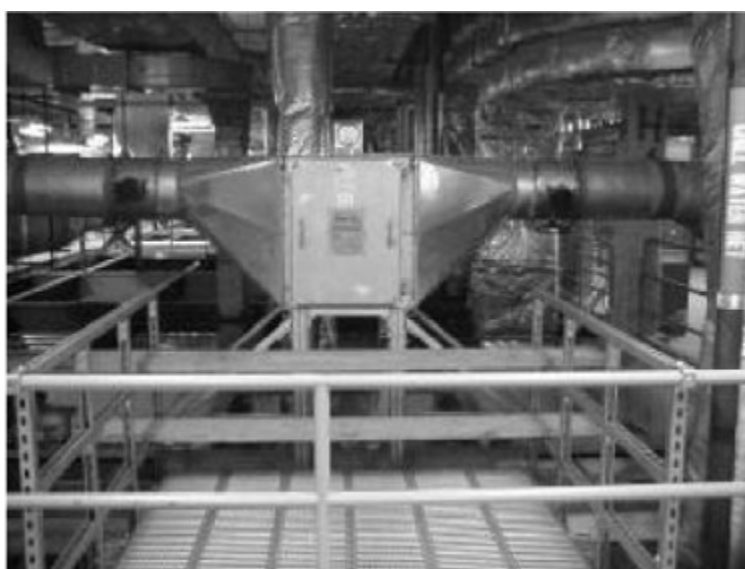
Figure 4.24: Correct Mounting of In-Duct-HEPA Filter Housing
