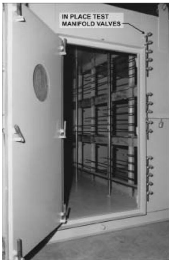
Figure 4.61: Filter Plenum Entry Door (No Airlock Type-Test Manifold with Valves Shown)
