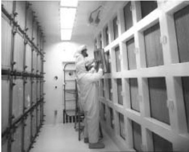
Figure 4.59: Blanking Plate Being Installed on Downstream Side of Mounting Frame
