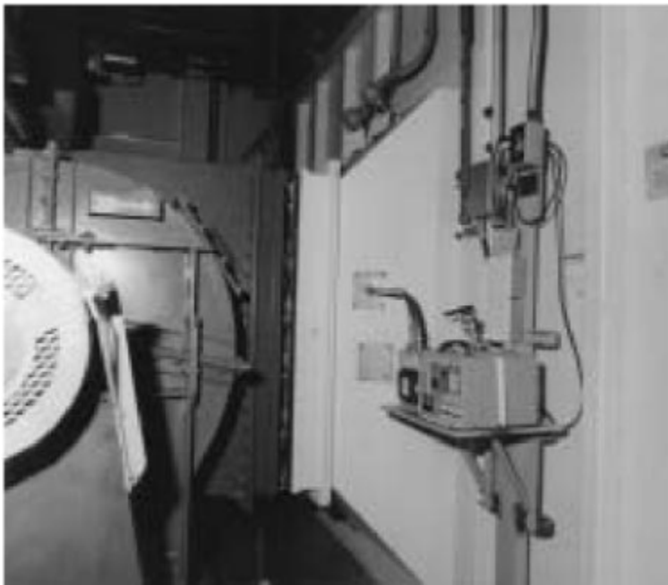
Figure 4.69: Air Monitor in Exhaust Duct from Plenum
